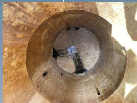
11-25-2023 Checking for dye in manhole
